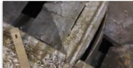
Traditional Structure After One Year of Use
